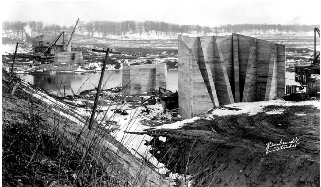
Photograph of early construction of the Staley Pump House
