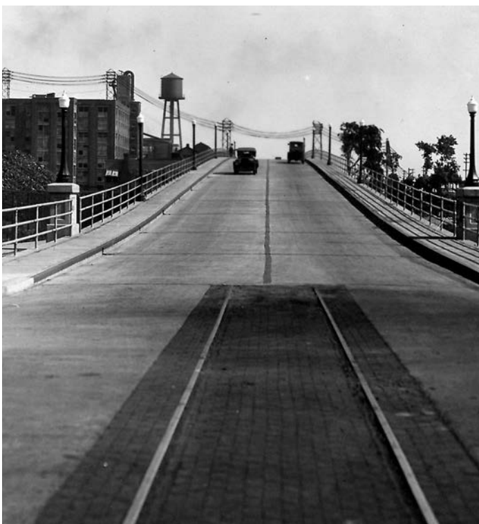
North-facing photograph of the newly built Staley Viaduct
