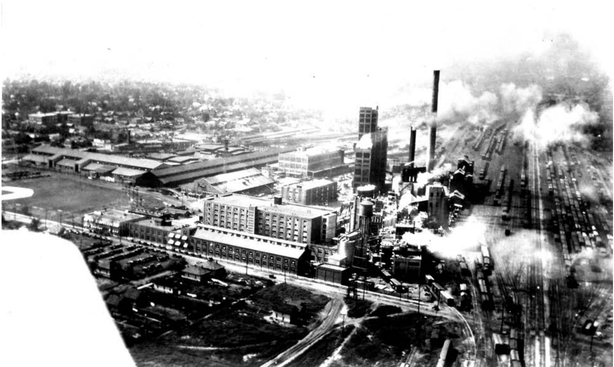
Photograph of the Staley Plant before the viaduct was built
