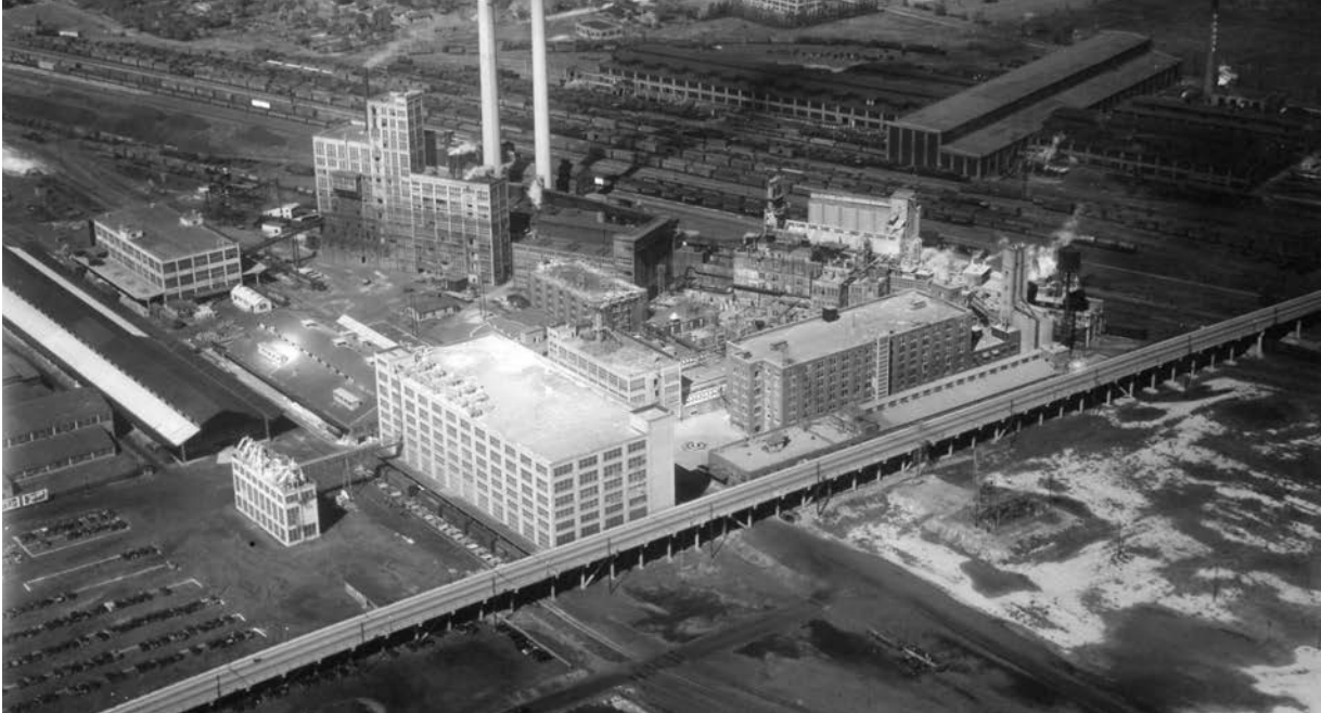
Aerial photograph of the Staley Viaduct
