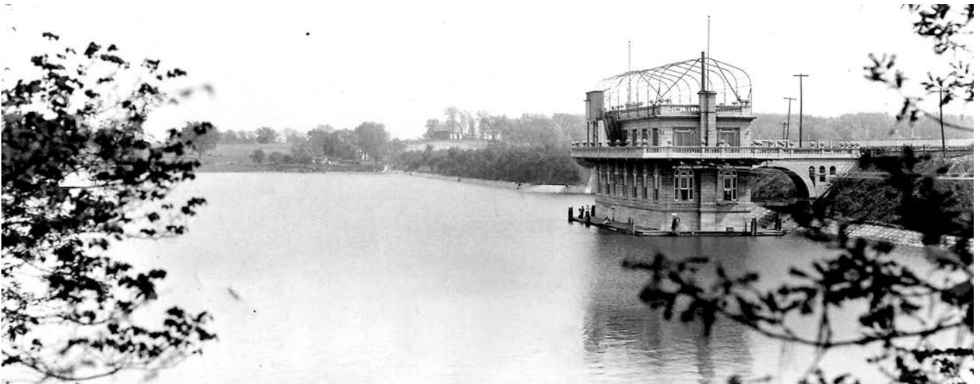
Photograph of the Staley Pump House on Lake Decatur
