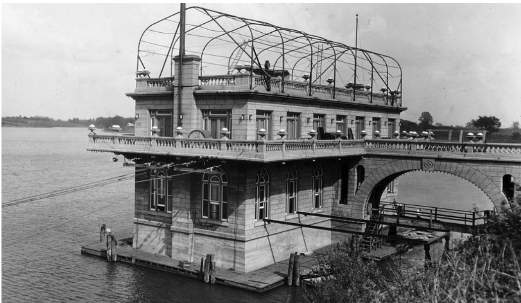
Photograph of the finished Staley Pump House
