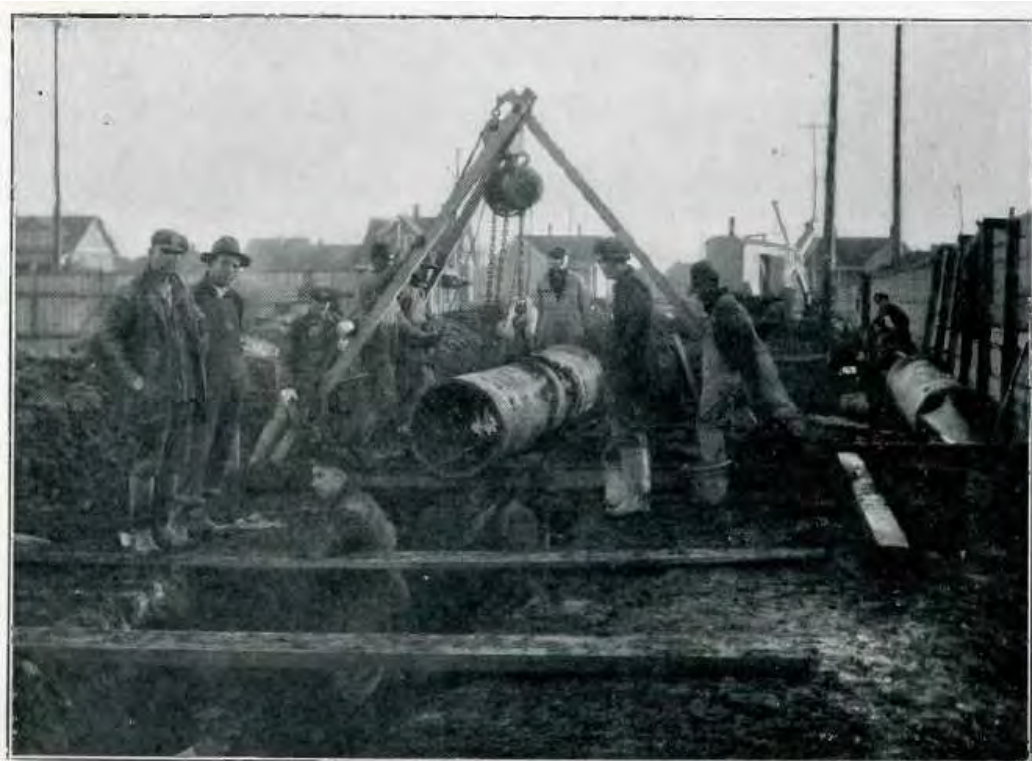
Figure 12. (Top) “Robinett and his affinity, the steam shovel, which digs the ditch for the water main from the river” ( Staley Fellowship Journal [December 1919], p. 3). (Bottom) “Laying the water main from the new pumping station. The quiet, mild appearing gentleman on the left is Zeke Coover, a caulking (corking) expert” ( Staley Fellowship Journal [December 1919], p. 3).
