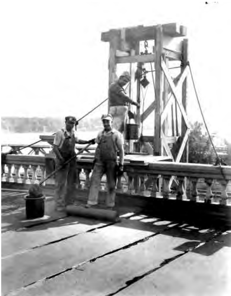
Figure 69. New tar roof being applied to the upper deck of the Staley Pumping Station and Club House, during renovation work of late 1944. By this time, the canopy had disappeared, and the use of the upper floor as a social space had been abandoned (Staley Museum). According to the Staley Journal , the use of the roof top of the Club House had been abandoned sometime ca. 1929 (“Work Starts on Renovation of Club House,” Staley Journal [October 1944], pp 25-26).
