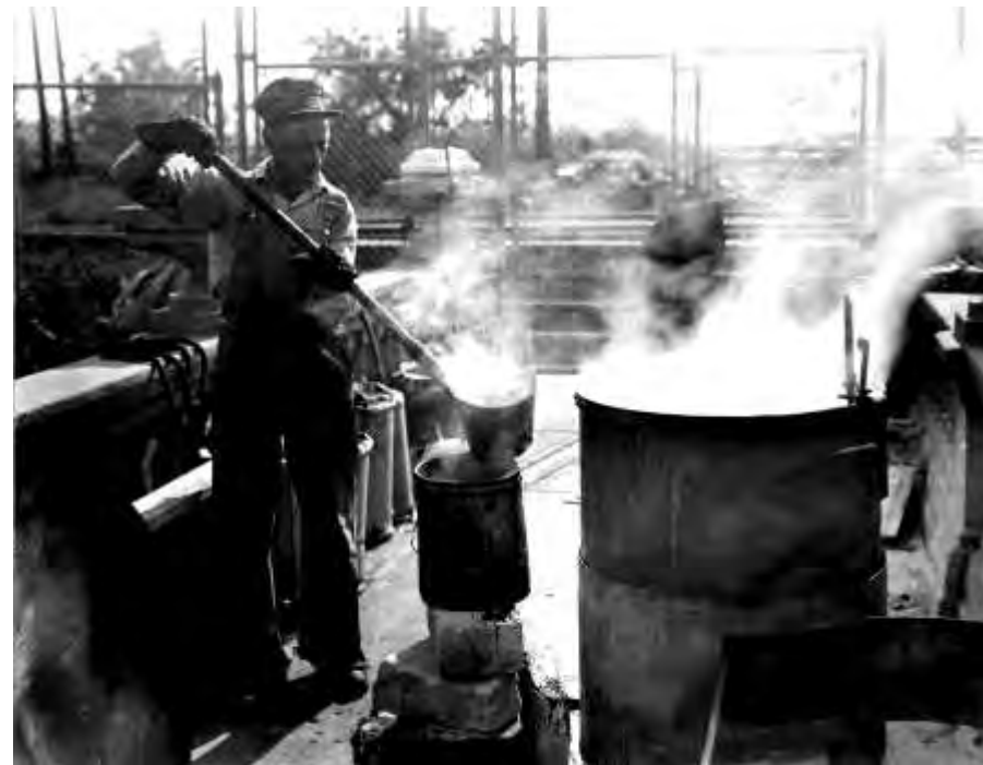
Figure 69. New tar roof being applied to the upper deck of the Staley Pumping Station and Club House, during renovation work of late 1944. By this time, the canopy had disappeared, and the use of the upper floor as a social space had been abandoned (Staley Museum). According to the Staley Journal , the use of the roof top of the Club House had been abandoned sometime ca. 1929 (“Work Starts on Renovation of Club House,” Staley Journal [October 1944], pp 25-26).
