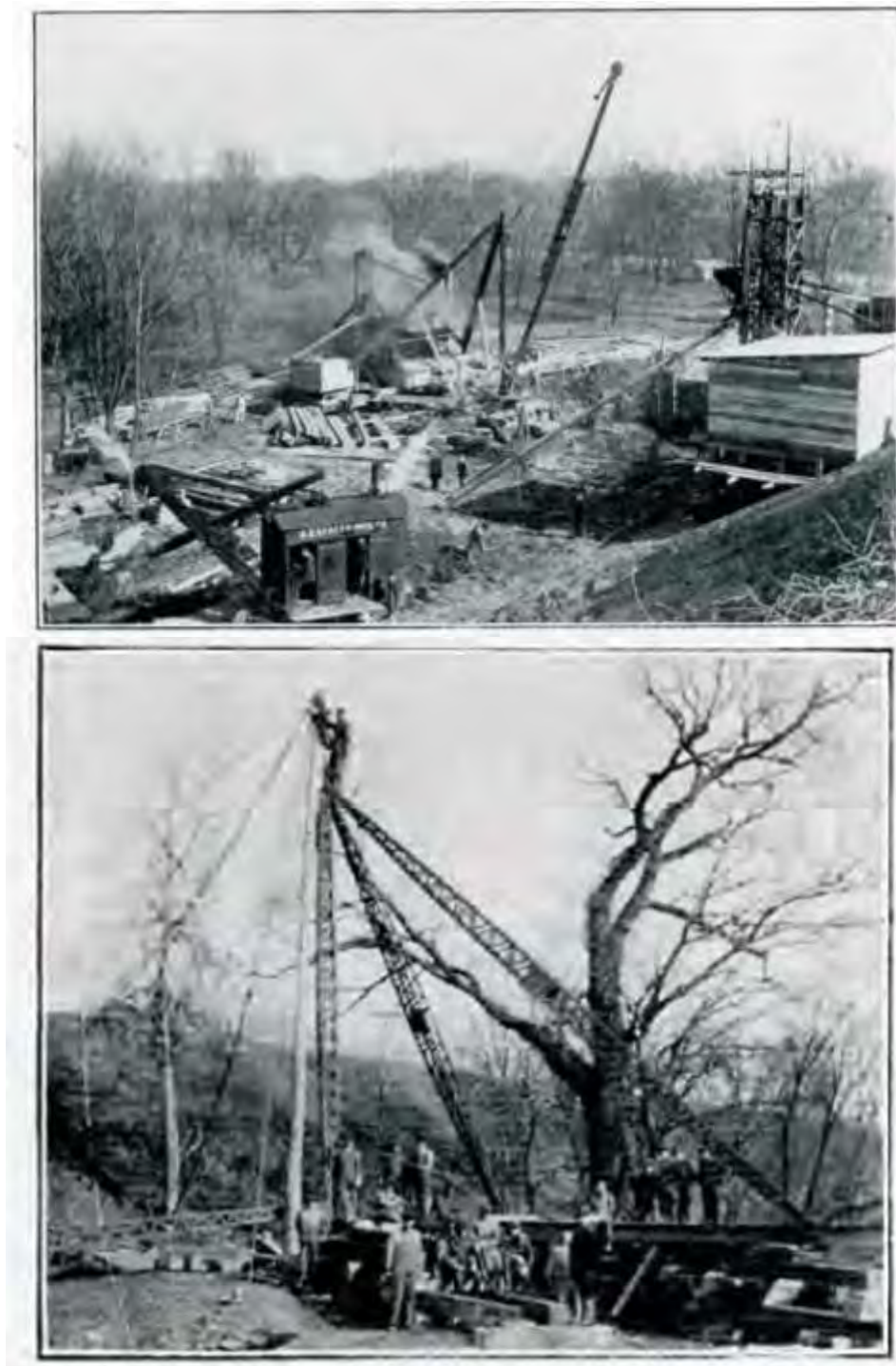
Figure 17. Two photographs of work at the Pumping Station ( Staley Fellowship Journal [April 1920], pp. 11, 17). (Top) “Showing the Steam Shovel Near the End of the Job of Digging the Ditch from the Plant to the Pumping Station.” (Bottom) “Beginning the Construction of Staleys Temporary Dam.” The temporary dam was located immediately to the south of, on opposite side of, the railroad trestle.
