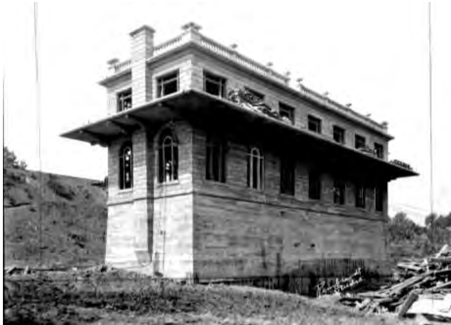
Figure 19. (Top) “The pumping station has finally crept this far above the surface of the ground” ( Staley Fellowship Journal [July 1920], p. 8). This photograph illustrates the scaffolding and wooden forms in place for the pouring of the concrete walls. (Bottom) “The Pumping Station which is rapidly nearing completion.” Southwest view of the building as illustrated in the October 1920 edition of the Staley Fellowship Journal ([October 1920, p.23; Staley Museum). The balustrade around the balcony had yet to be installed at this point. The opening in the roof-line balustrade marks the point to which the exterior stairway was aligned.
