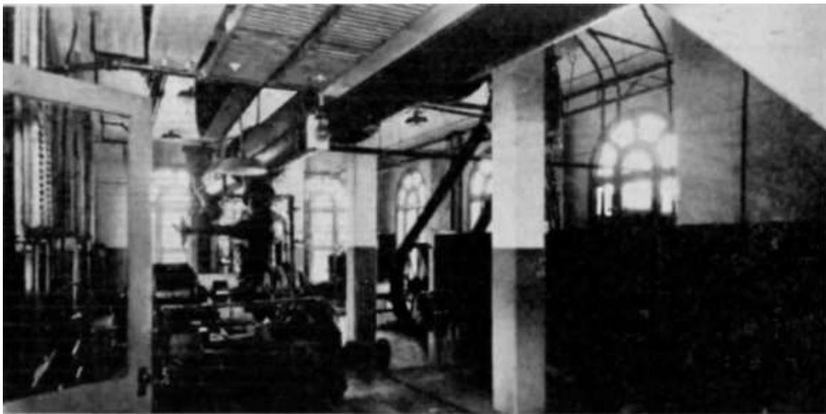
Figure 55. Two early views of the interior of the Staley Pump House, illustrating the interior of the pump room (or “landing”) level of the building (Watson 1923:6). (Top) “First Floor Pumping Station—The two 100 H. P. pumps in the foreground. Intake valves in background.” (Bottom) “First Floor Pumping Station—West End, 150 H. P. pump in foreground.”
