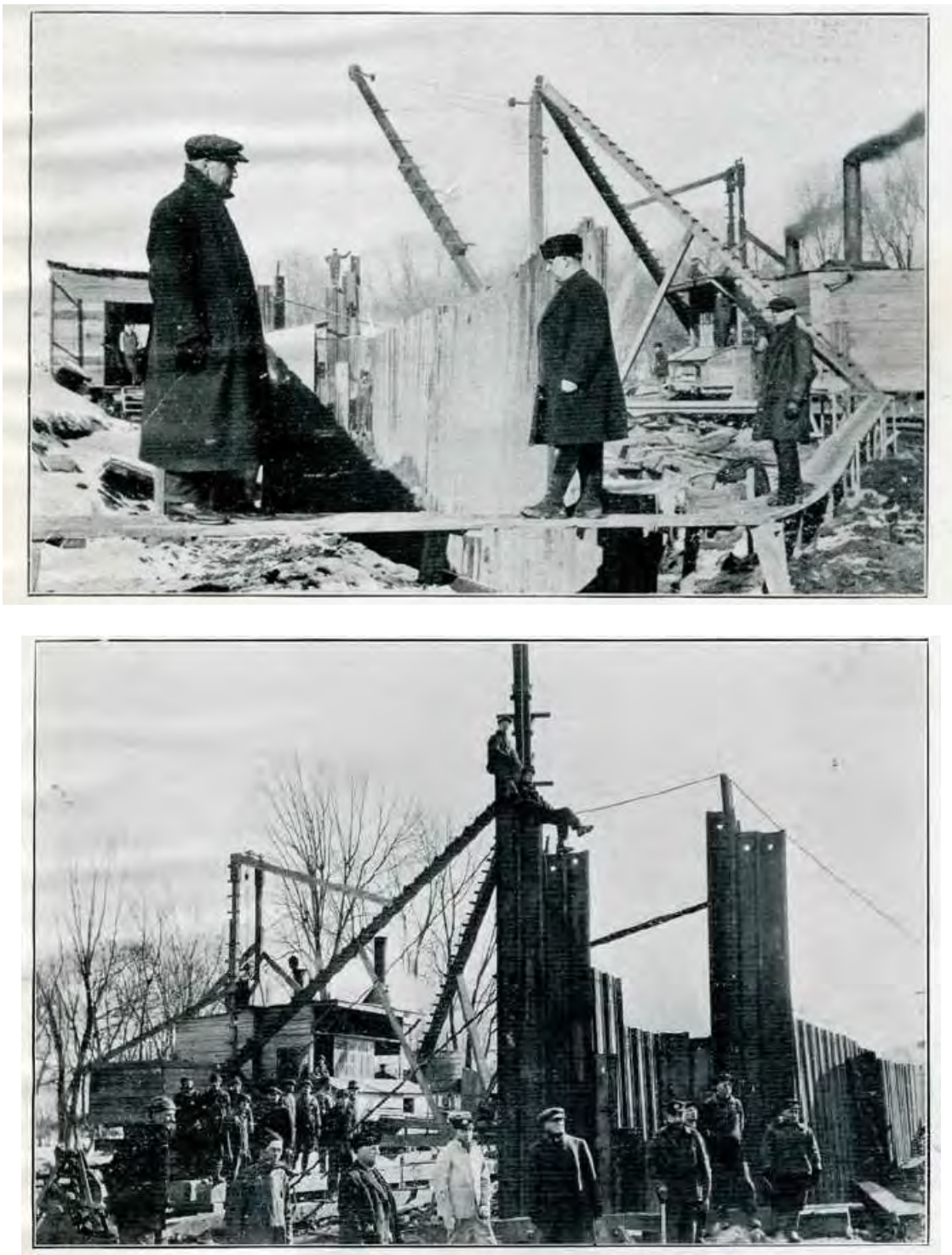
Figure 18. (Top) “A winter scene along the banks of the Sangamon” ( Staley Fellowship Journal [February 1920], p. 5). (Bottom) “Driving the last sheet of steel bulkhead for the 36-inch intake from the river” ( Staley Fellowship Journal [February 1920], p. 9).
