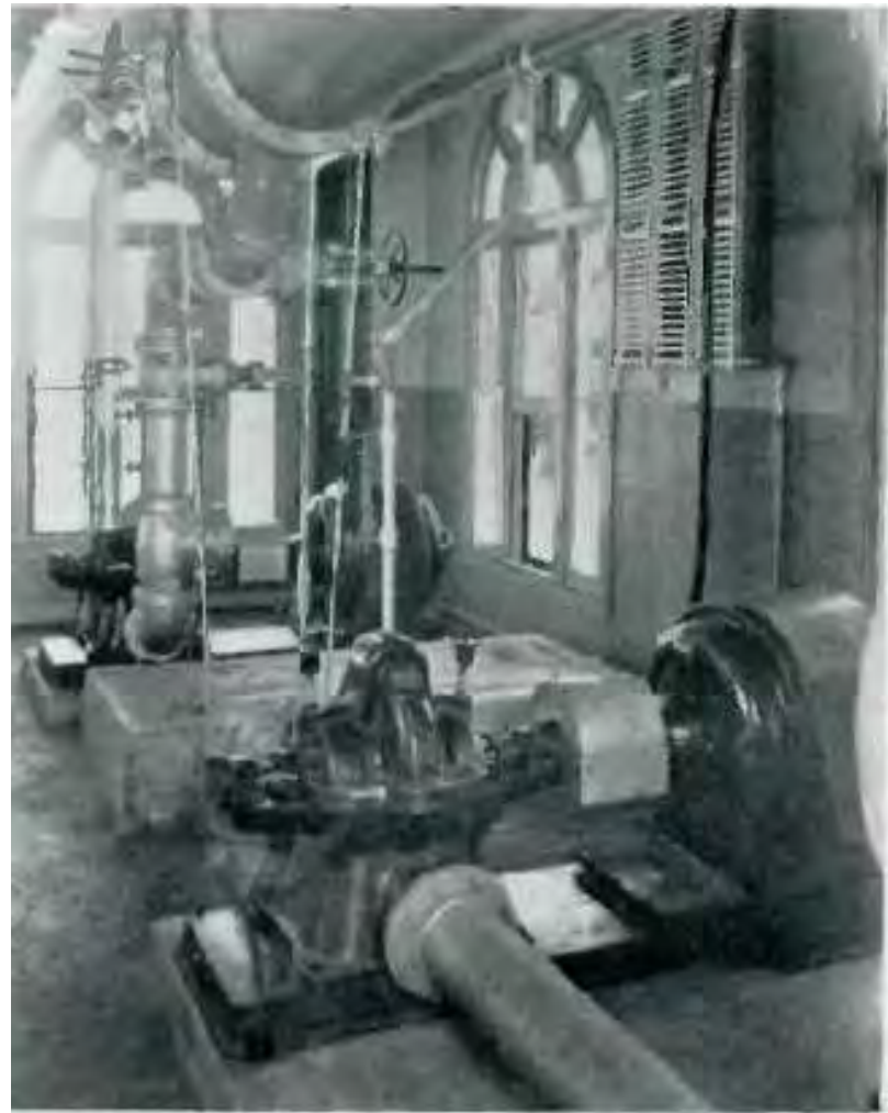
Figure 61. (Left) “Henry Meyer polishing the deep well pump.” (Right) “A and B pumps at the south end of the pump room” ( Staley Journal [September 1938], p 5).
