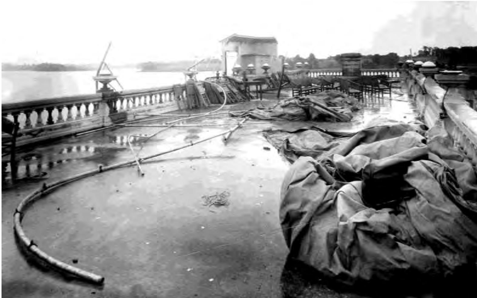
Figure 41. View of Roof Level illustrating storm damaged canopy and a couple of lamp globes (looking east). Note frame toilet structure at the far end, adjacent to the stair landing (Undated [ca. 1929] photograph; Staley Museum).
