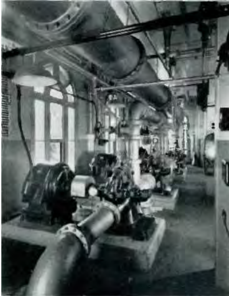
Figure 62. (Left) “These four pumps, C and D units, are in almost continuous service.” (Right) “The hoisting mechanism shown here raises and lowers the screens between the intake and suction chambers in the level below this shown” ( Staley Journal [September 1938], p 5).
