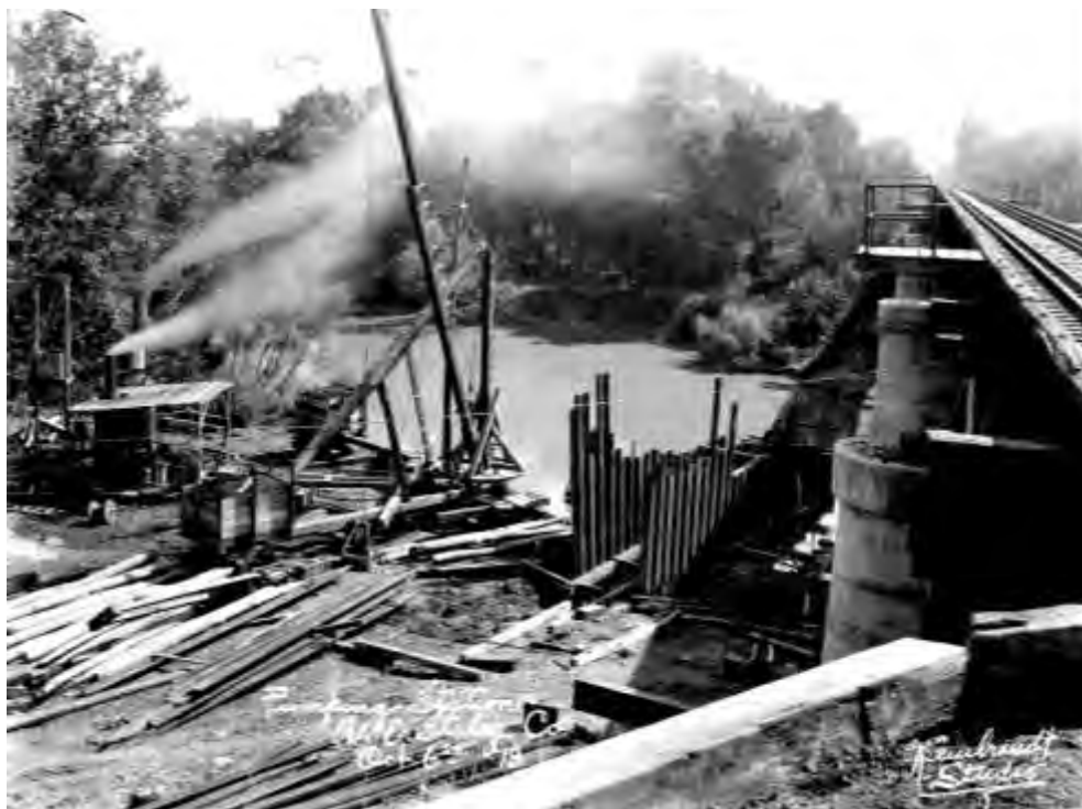
Figure 11. Two views of work on the intake pipe to the Pumping Station, both dated 6 October 1919. The bottom image was published as “View of Work on Pumping Station from the I. C. Tracks” (Staley Museum; Staley Fellowship Journal [November 1919], p. 14).
