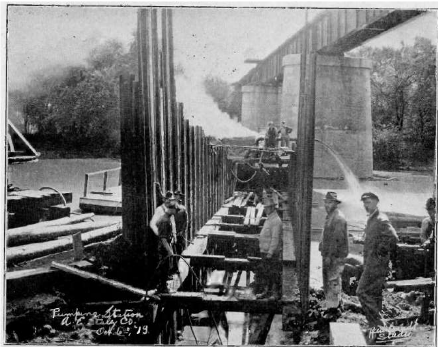
Figure 10. (Top) Photograph labeled “Pumping Station” and dated March 1920, illustrating work on the intake pipeline and/or water line along Sangamon River (Staley Museum). (Bottom) Photograph Labeled “Pumping Station,” dated October 1919, with caption that read “The coffer dam which permits laying the large intake pipe to the pumping station many feet below the surface of the water” ( Staley Fellowship Journal [November 1919], p. 17).
